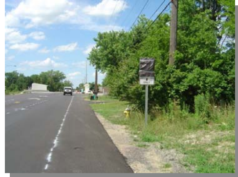
North Dixie Drive Before Improvement
