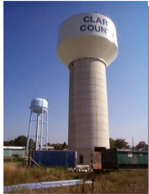
1,000,000 gallon water tank in Clark County
