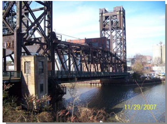
Columbus Road Lift Bridge Looking West
