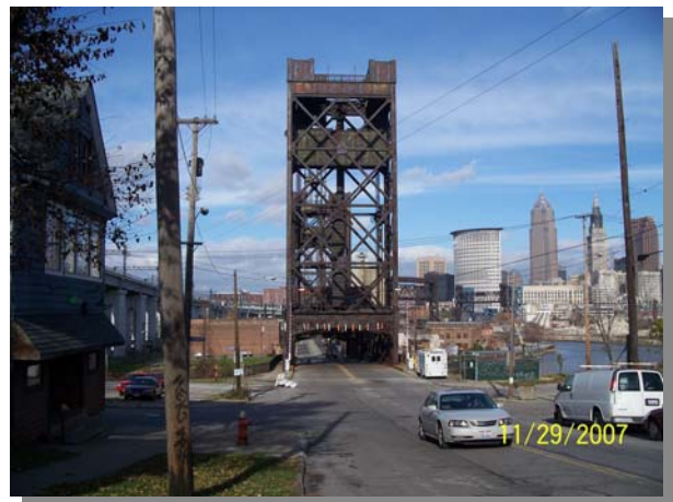
Columbus Road Lift Bridge Looking North
