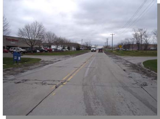
Trolley Industrial Drive – East Before Construction
