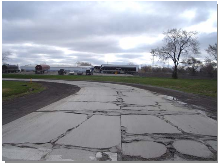
Trolley Industrial Drive – East Before Construction
