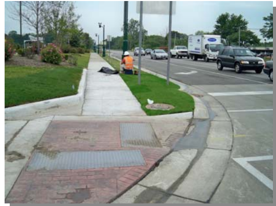
Ford Road Turn Lane and Ramp Installation (After Construction)
