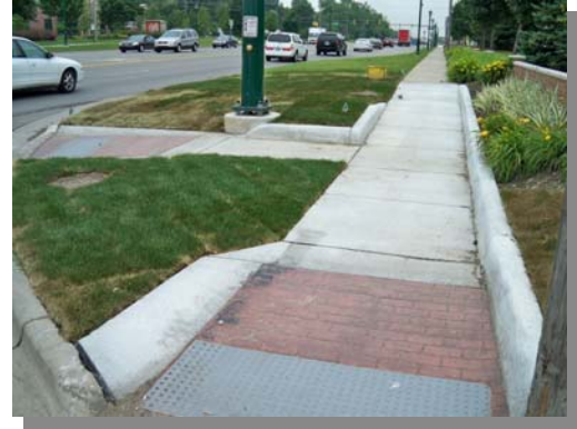
Typical ADA Sidewalk Ramp Installation (After Construction)
