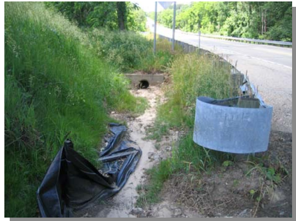
Concrete Culvert on South Side of US-12 – Before Construction
