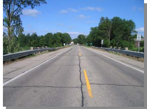
US-12 Bridge B01 Before Construction
