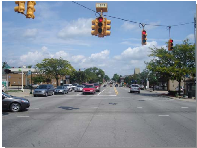
M-150 Before Construction
