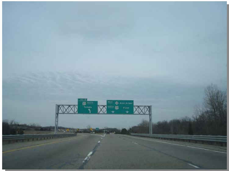
M-14 Cantilever Sign Before Improvement
