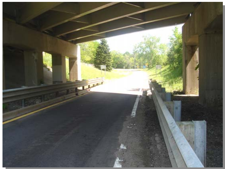
I-94 EB Exit Ramp to I-94BL (Before Construction)
