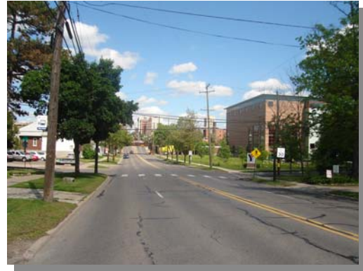
I-94BL Approaching Downtown Ann Arbor (Before Construction)
