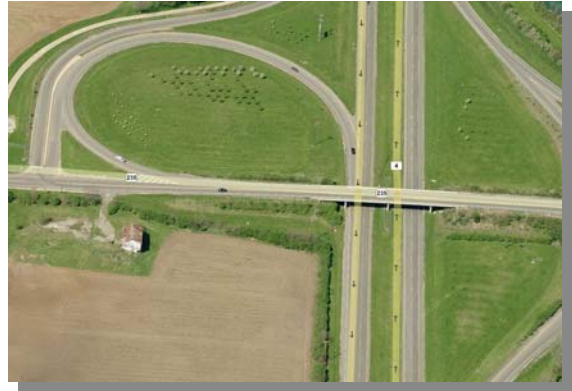
MOT-235 Before Construction
