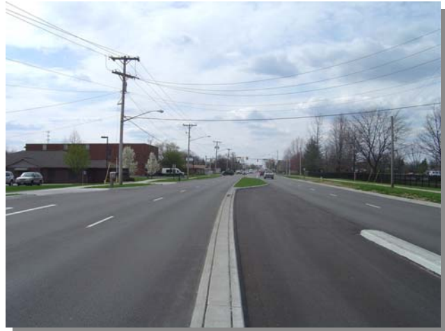
Dayton Yellow Springs Road After Construction
