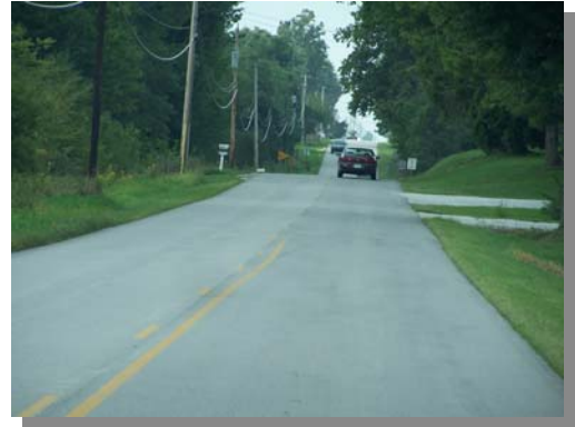
CR 300 Looking West Before Construction
