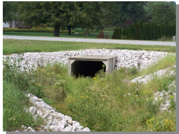
Culvert Passing Under SR 26 Before Construction
