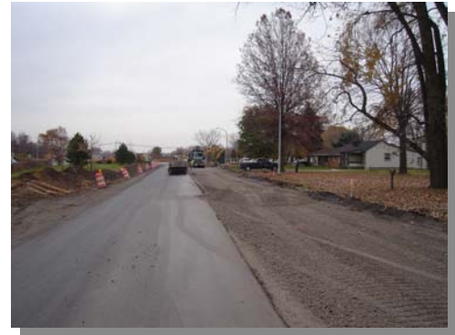
Holland Road during Construction
