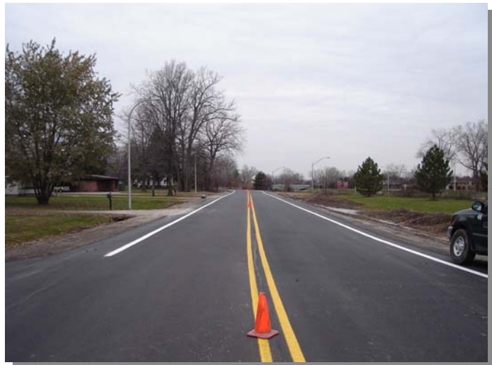
Holland Road during Construction
