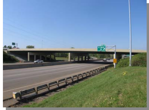
South Main Street over I-277
