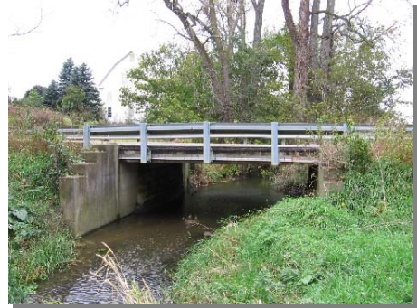
CHP-559-0165 – Existing Structure
