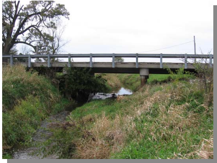
CHP-599-0691 – Existing Structure
