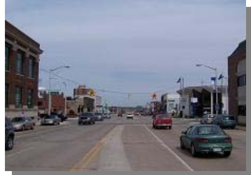
I-94 BL – Existing Condition
