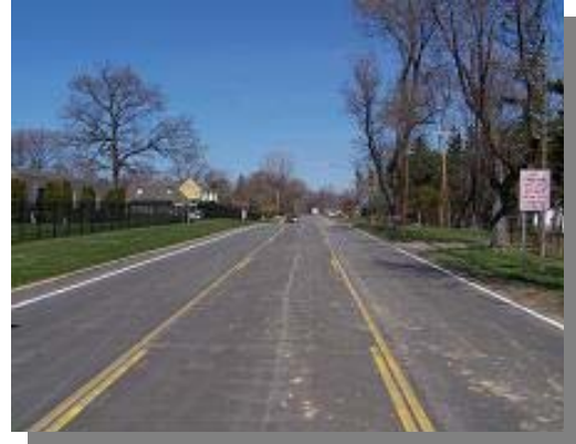
I-94 BL – Existing Condition
