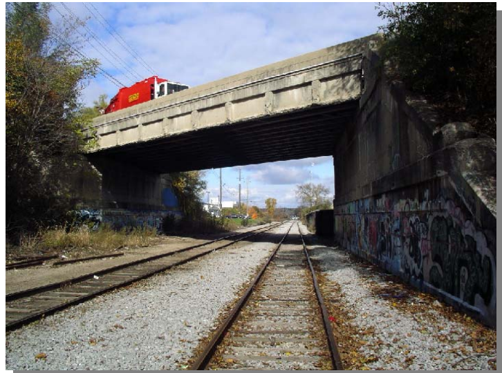
Stadium Boulevard over Ann Arbor RR – Existing Bridge
