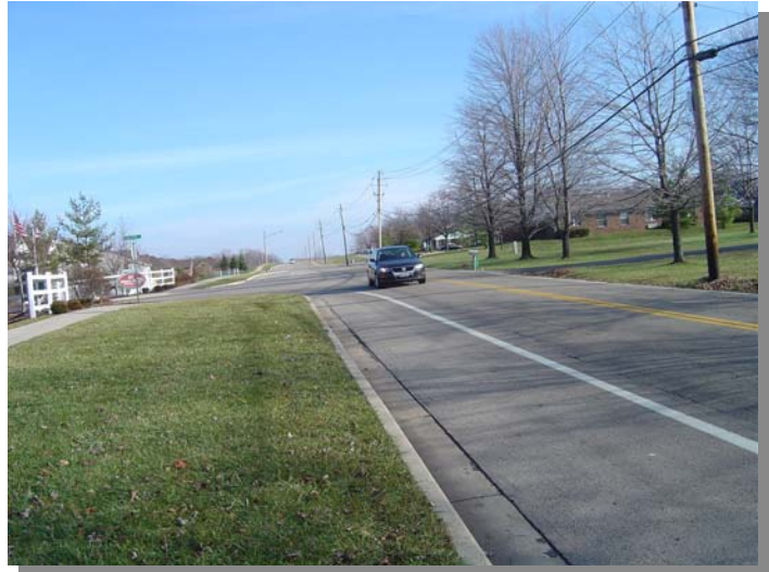
Spring Valley Pike Before Construction
