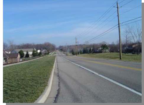
Spring Valley Pike Before Construction
