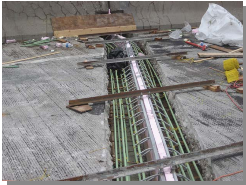
M-20 over CSX RR New Expansion Joint
