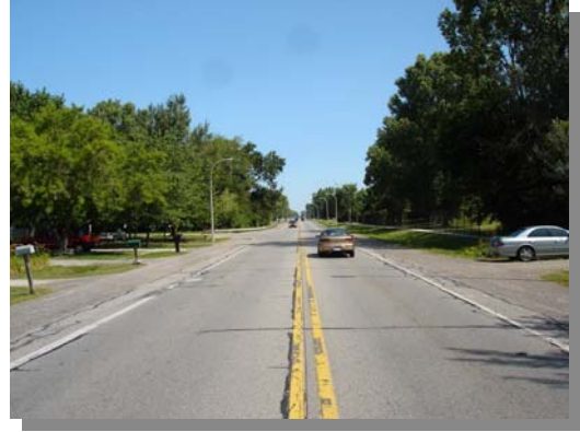
Beech Daly Road Before Construction
