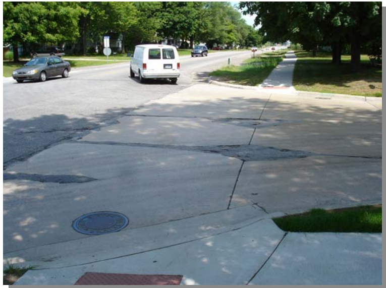
Beech Daly Road Before Construction
