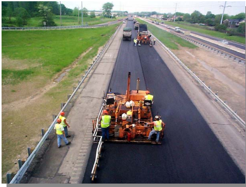
Paving EB Lanes
