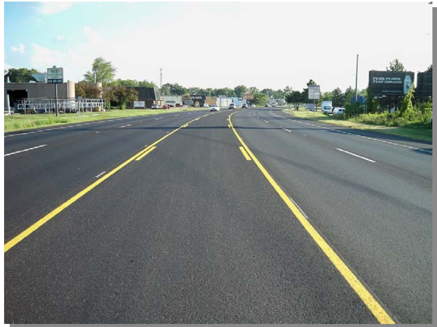
M-97 Southbound After Construction
