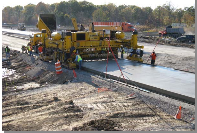
Concrete Paving on Northbound M-85 Ramp from I-75
