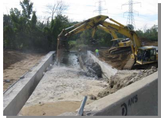
Silver Creek Box Culvert Removal
