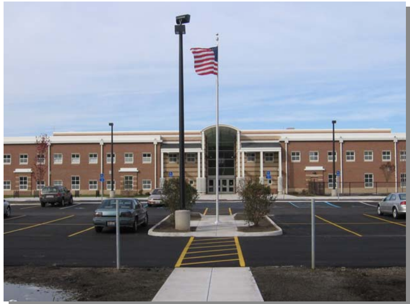
Reynolds Elementary Front Entrance and Main Parking Lot
