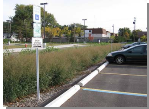
Faculty & Staff Parking Lot Bioretention Cell
