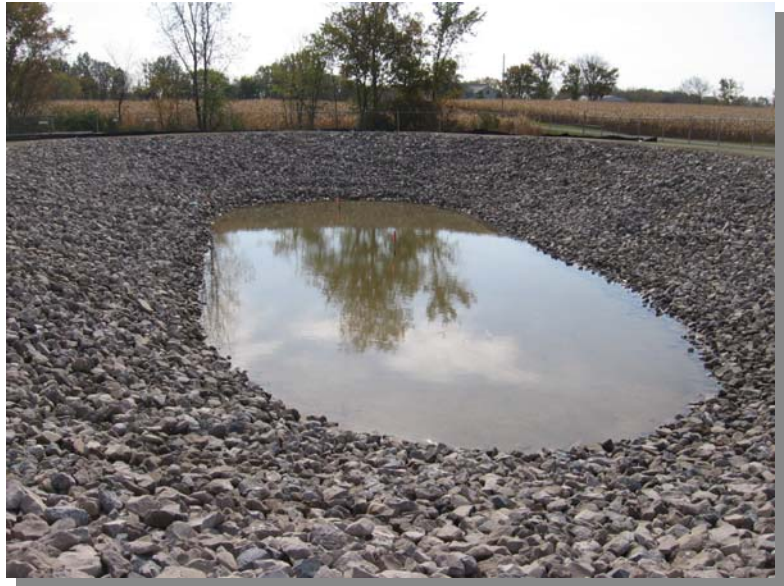
Wastewater Lagoon Improvement
