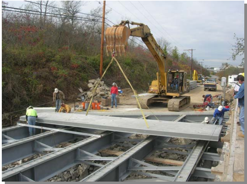
Placement of FRP Deck
