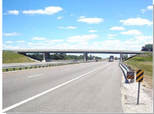
Tracy Road over Ohio Turnpike
