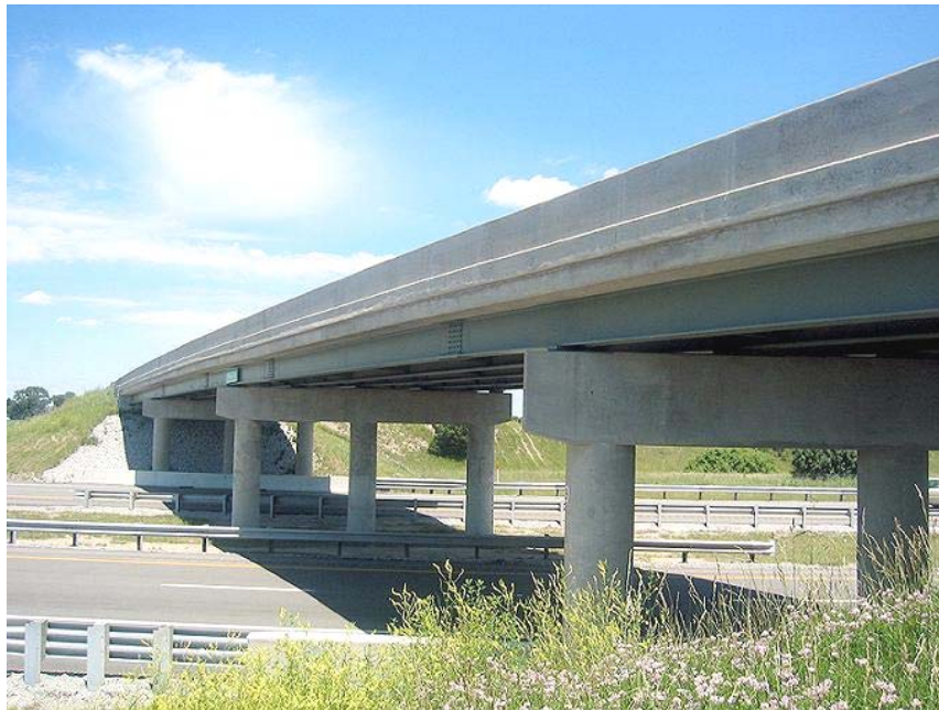
Tracy Road over Ohio Turnpike
