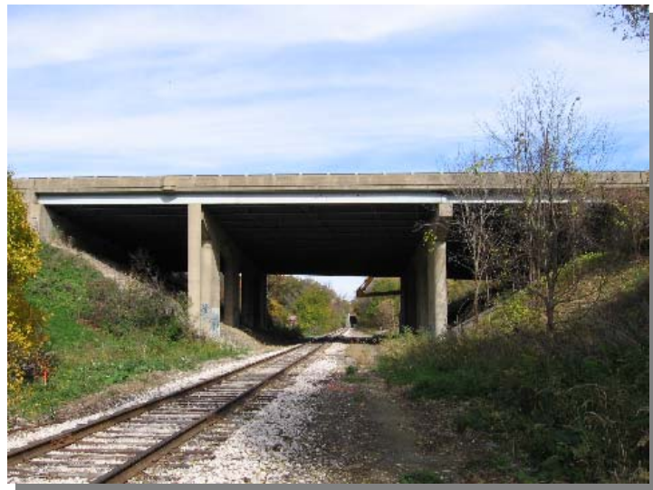
MAH-680-0693 – Existing Structure
