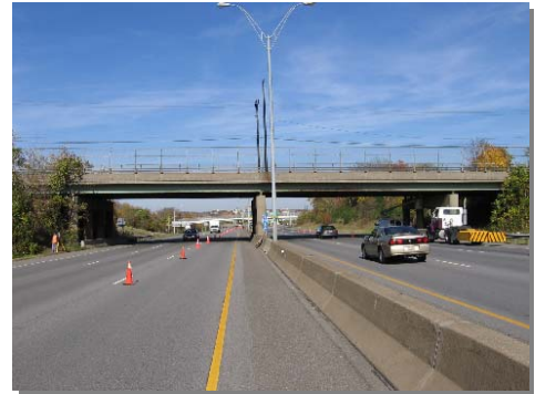
MAH-62-1751 – Existing Structure
