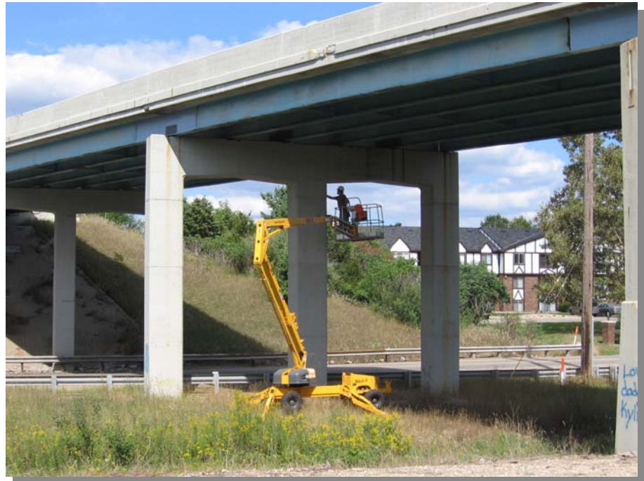
US-131 over Amtrak and KL Ave.
