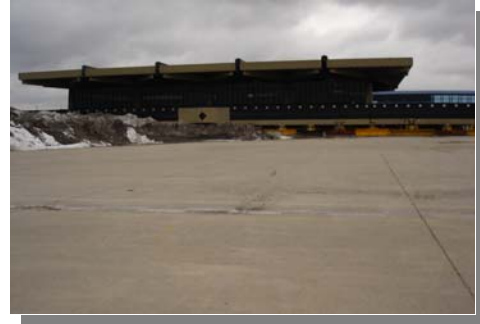
Existing J.M. Davey Terminal (North Terminal) and Apron
