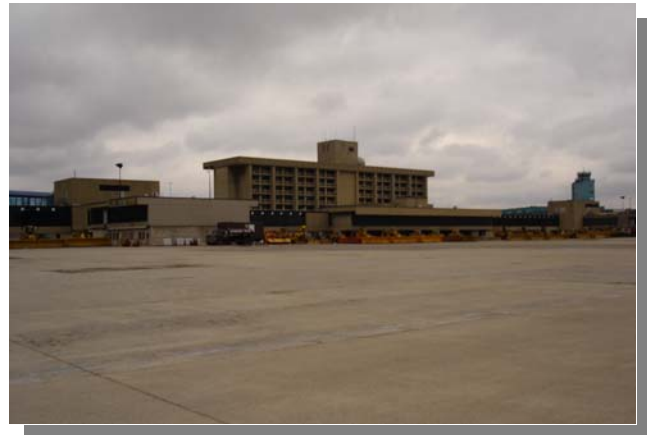
Existing Control Service Building (Marriott Hotel) and Apron
